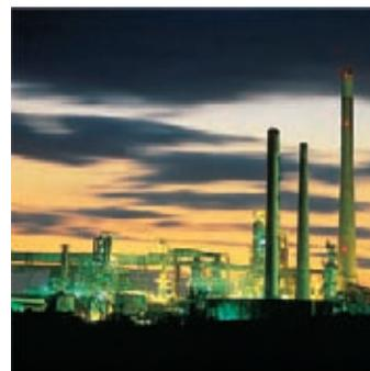
**Petroleum refinery.** The towers contain catalysts that break up large molecules in hot crude oil to smaller molecules suitable for vehicle engines. (*Martin Bond/Photo Researchers*)
